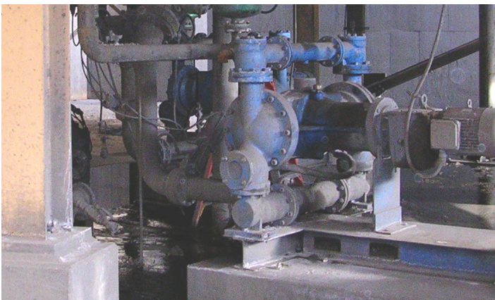
EM Pump as Thickener Underflow Pump
