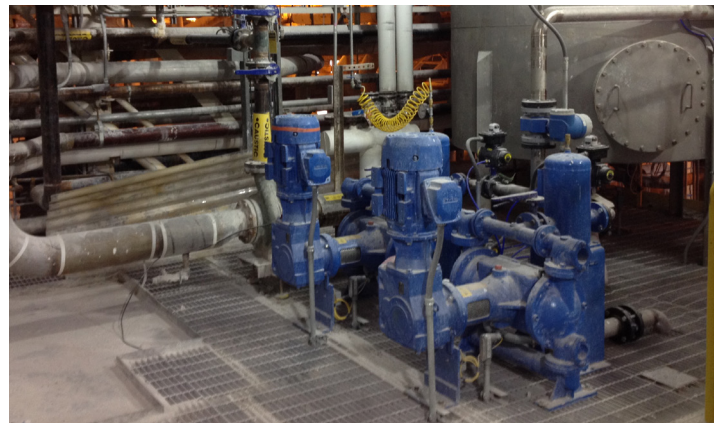
Bevel gears with vertically mounted electric motors provide space saving installation.
